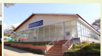
Industrial Scale Enzyme Bioprocessing Facility
