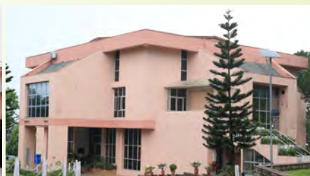
Library and Auditorium
